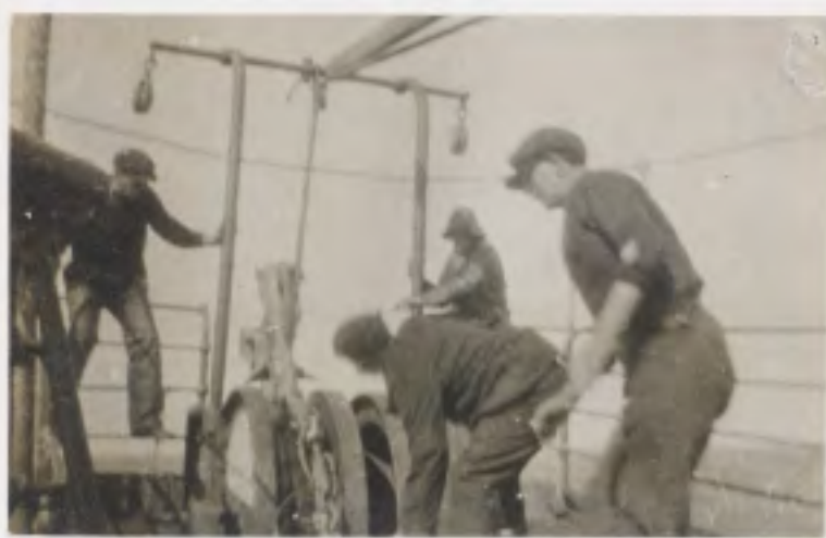
3. Getting a Lucas cutting Grapnel on board.
