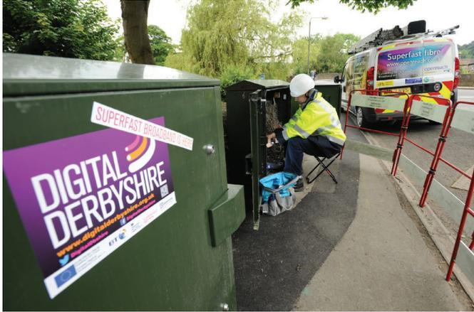
Twenty green roadside fibre cabinets have been installed in the town and more than 25km of fibre cable laid underground as part of the work.
